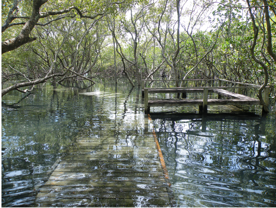
Figure A1. Submerged boardwalk at Ukerabah historic site, Tweed Heads. Photo: Lance Tarvey, DECCW.
