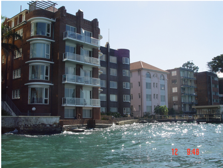
Figure A11. Limited freeboard to crest of foreshore revetment structures at Kirribilli Point, Sydney Harbour. Photo: Adrian Turnbull, North Sydney Council.
