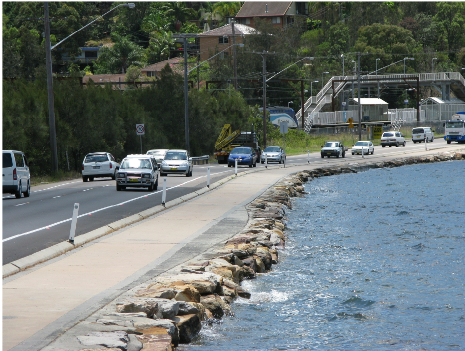
Figure A7. Limited freeboard to crest of foreshore revetment along Brisbane Water Drive, Tascott, Brisbane Water. Photo: Phil Watson, DECCW.
