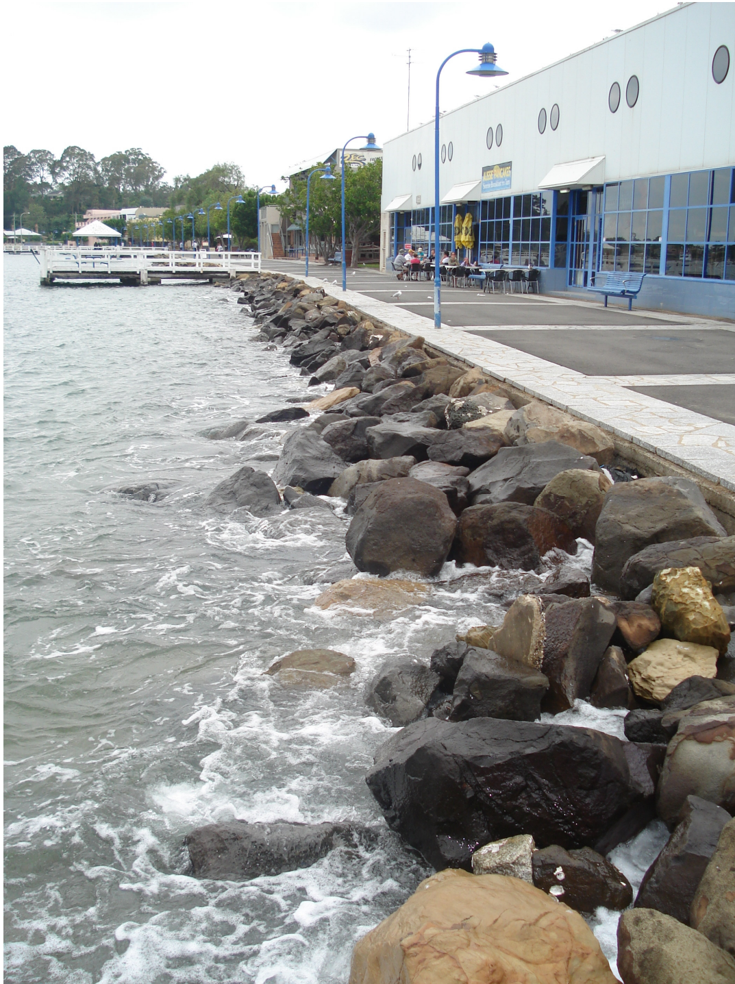
Figure A15. Limited clearance to top of seawall along foreshore at Batemans Bay, CBD. Photo: Lindsay Usher and Norm Lenehan, Eurobodalla Shire Council.
