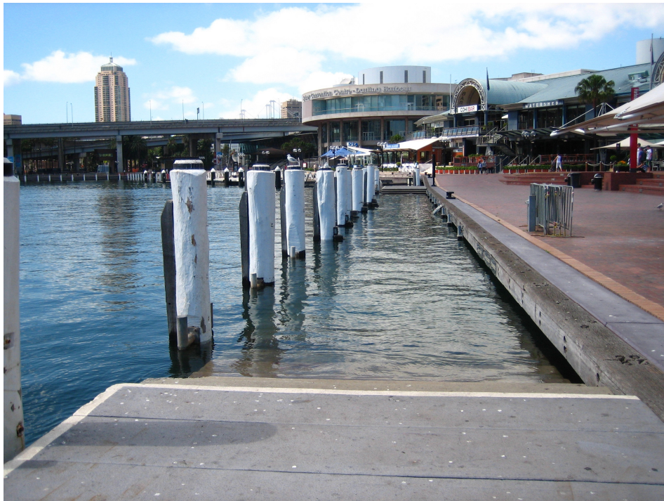
Figure A12. Limited freeboard to hardstand walking areas at Harbourside, Darling Harbour. Photo: John Gan.
