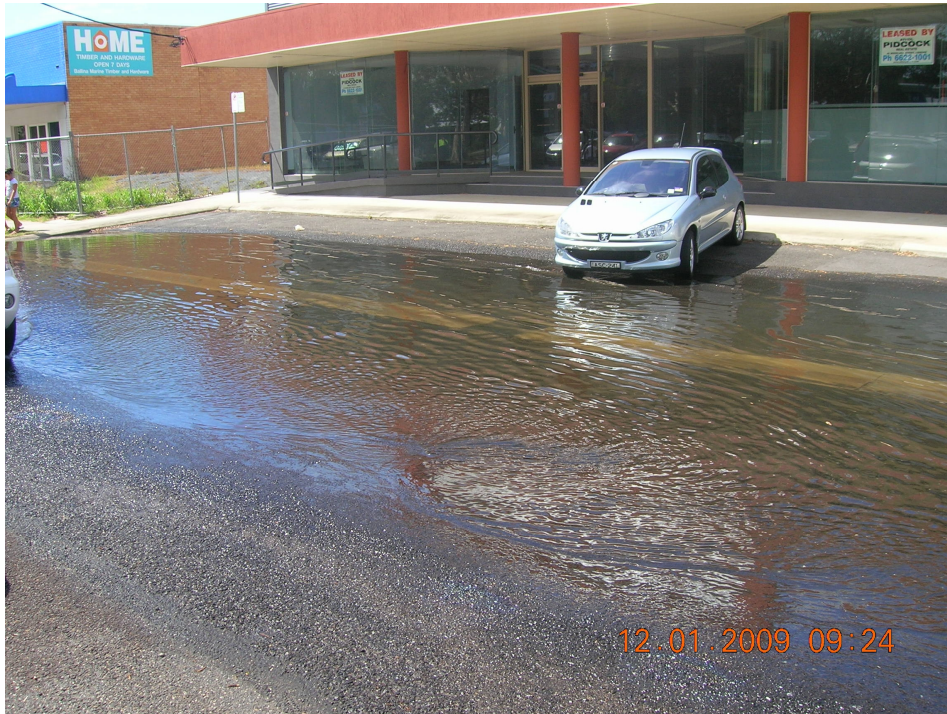
Figure A3. Tidal waters of the Richmond River penetrating back up through the stormwater system at Tamar Street, Ballina. Photo: Ballina Shire Council.
