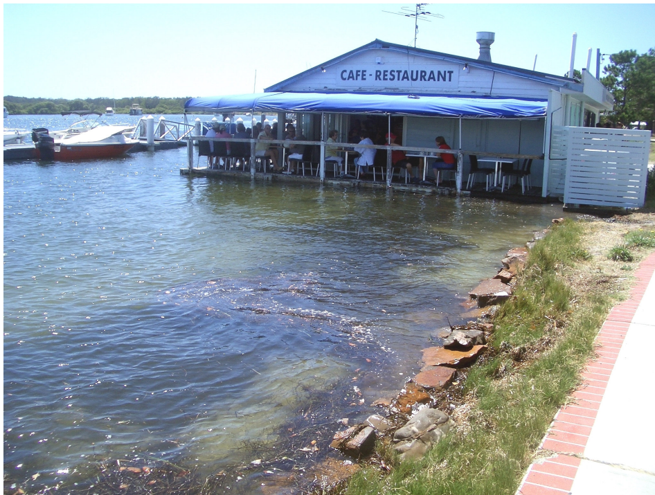
Figure A6. Tidal waters lapping at the ground floor level of the Boat Shed Café, Tea Gardens, Myall River. Photo: Kevin Haskew.
