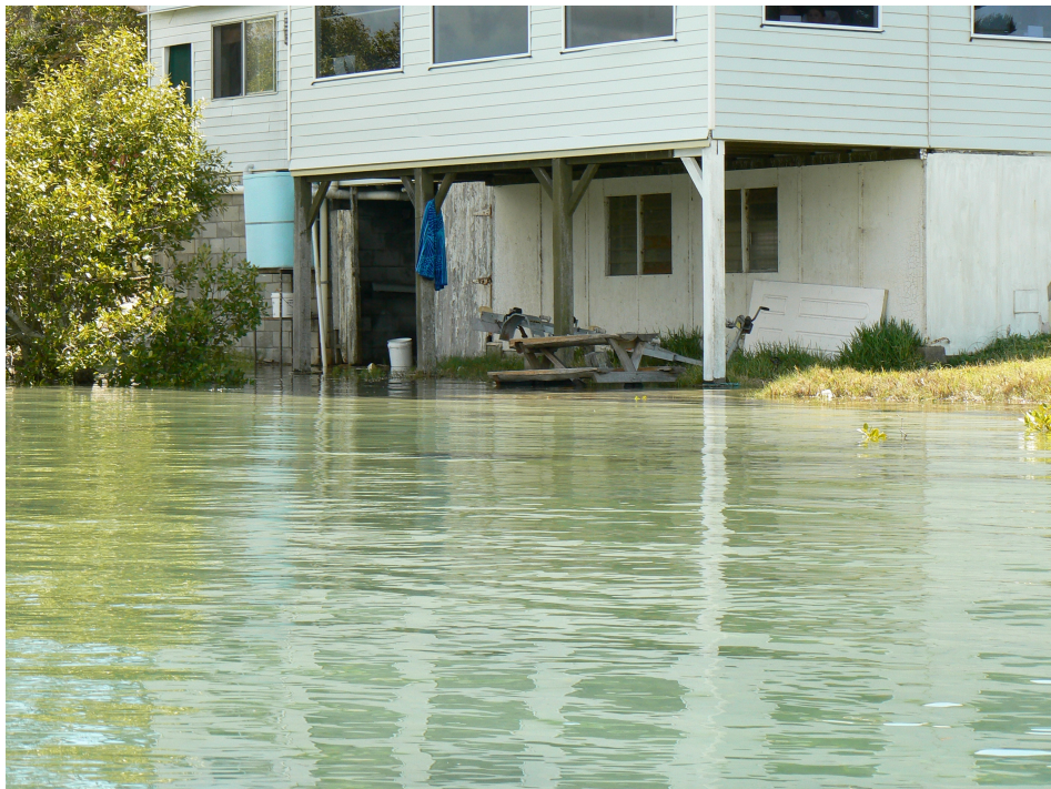
Figure A4. Tidal waters of the Wooli Wooli River penetrating into the rear of the Wooli Kiosk, River Street, Wooli. Photo: Wayne Jubb.
